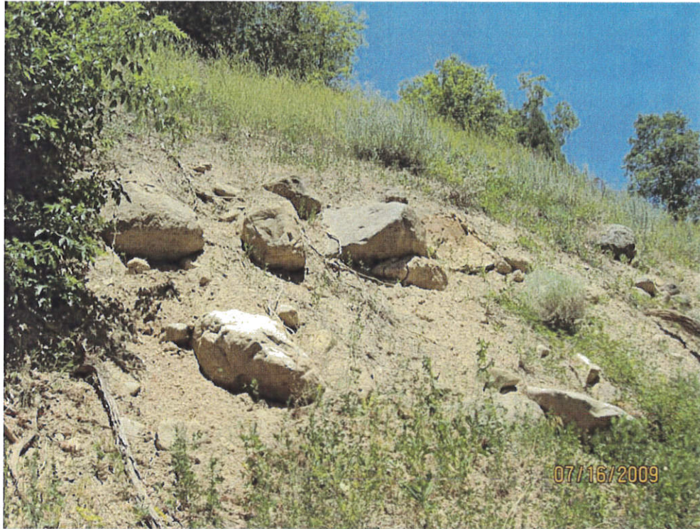
Loose rock exposed in high wall just north of Ogden Canyon Canal Conduit, northeast of property
