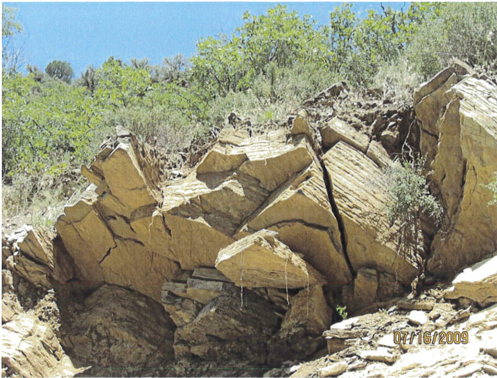
Fractured rock outcrop located just north of Ogden Canyon Canal Conduit
