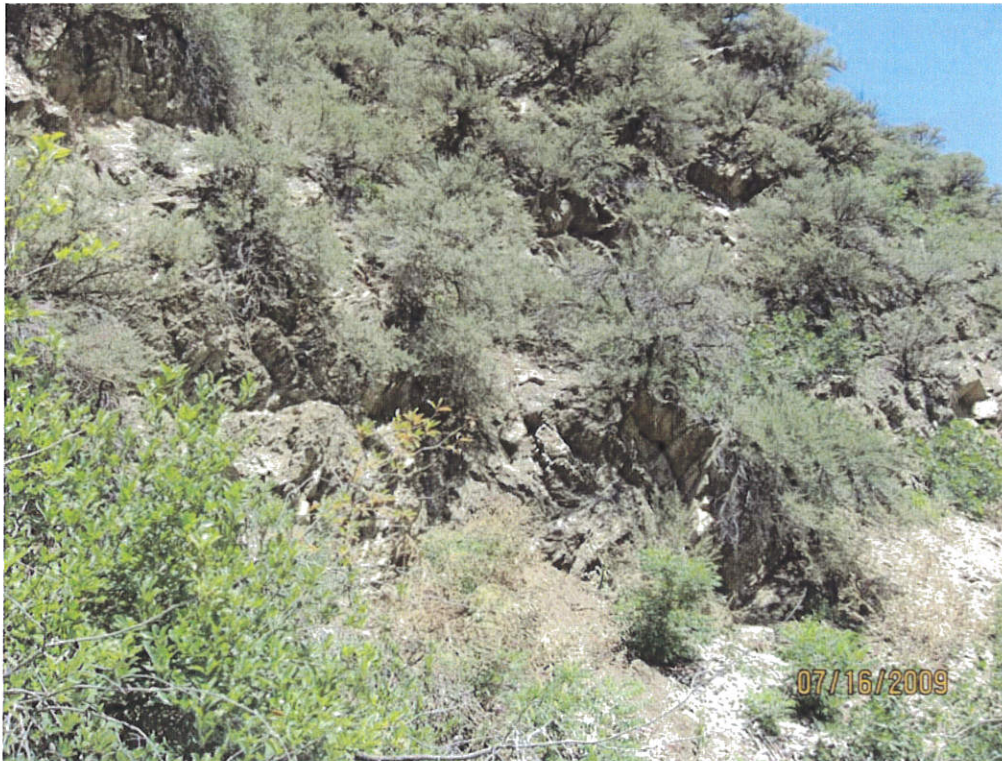
Typical rock outcrop exposed just north of the Ogden Canyon Canal Conduit above the property
