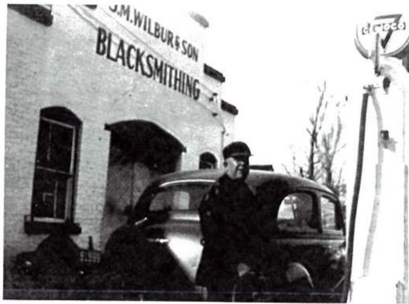
Exhibit D: Original Blacksmith Shop Architectural Detail
