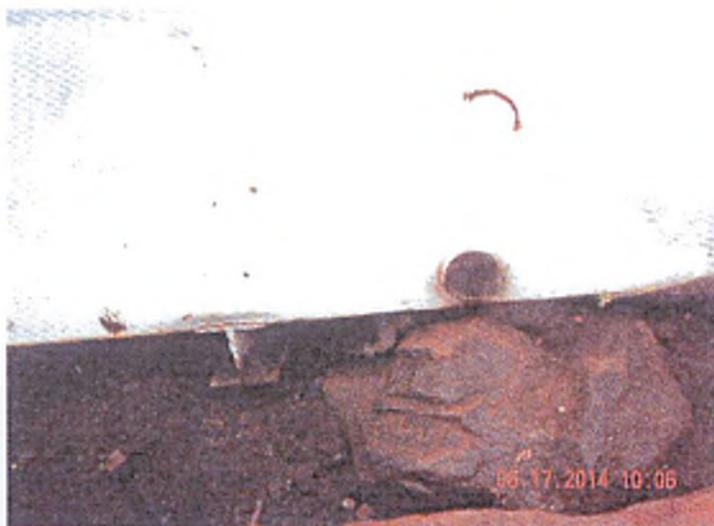
Fuel storage tank secondary containment with missing drain plug
