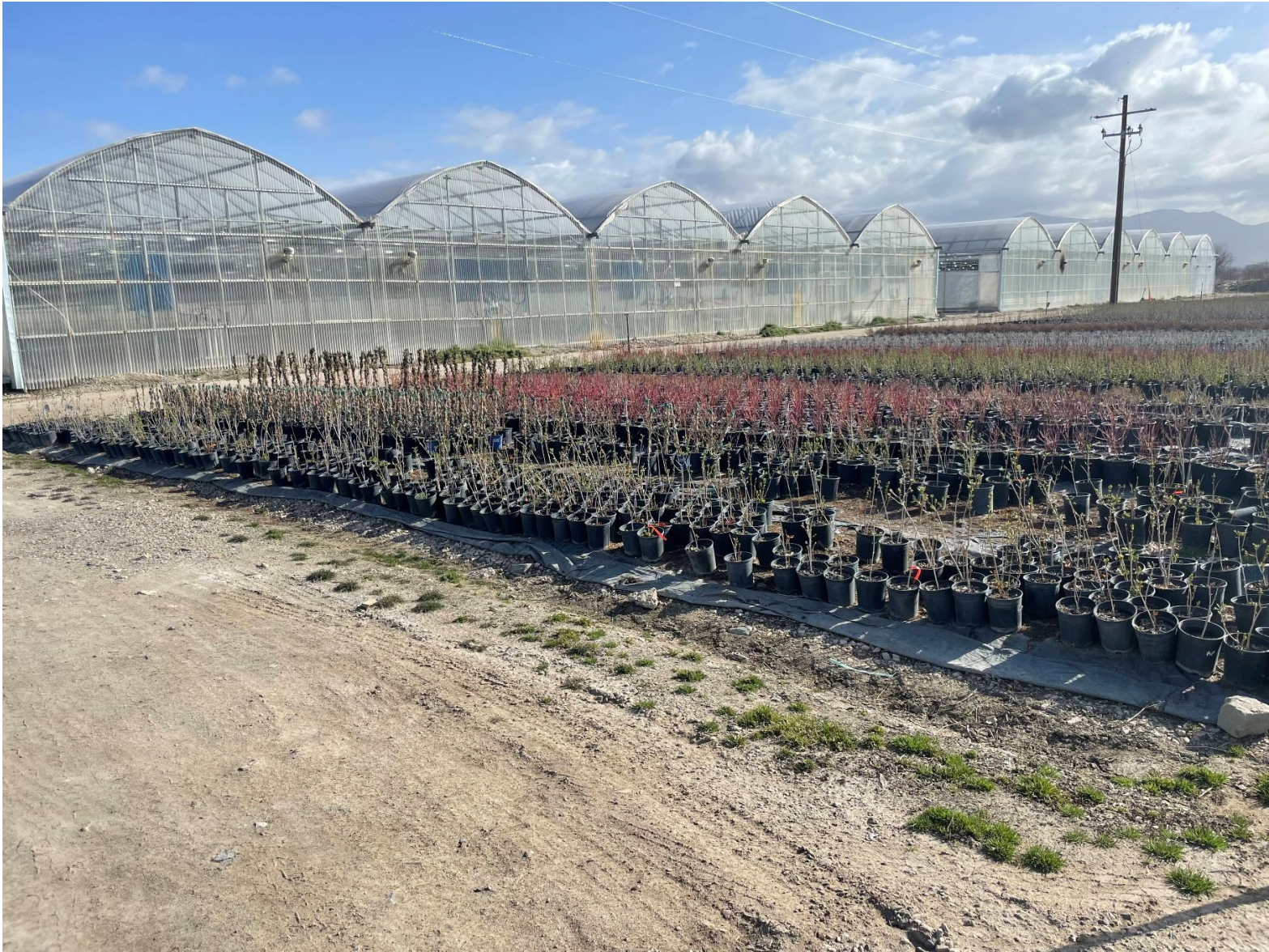
S-3, S-4, and S-4 EXTENTION GREENHOUSES PHOTO
