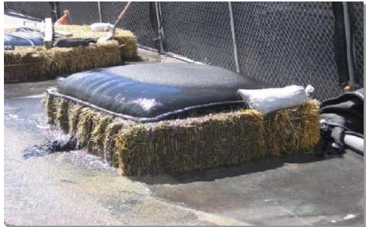
Photograph DW-1. A relatively small dewatering operation using straw bales and a dewatering bag.
