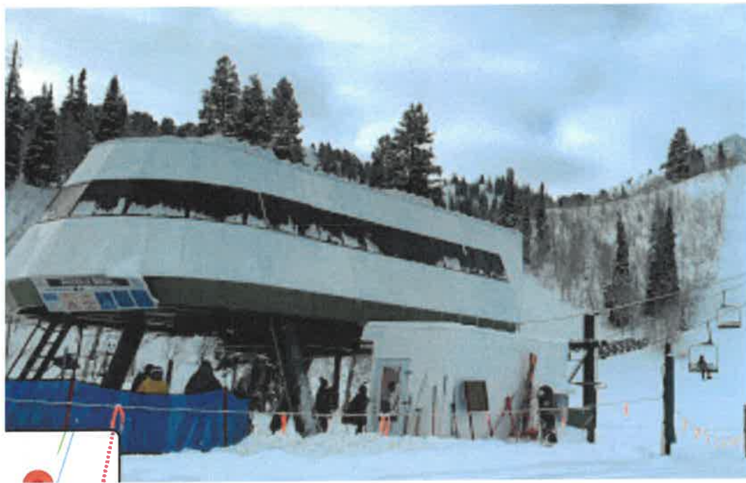
Current lift terminal at the bottom of Middle Bowl.
