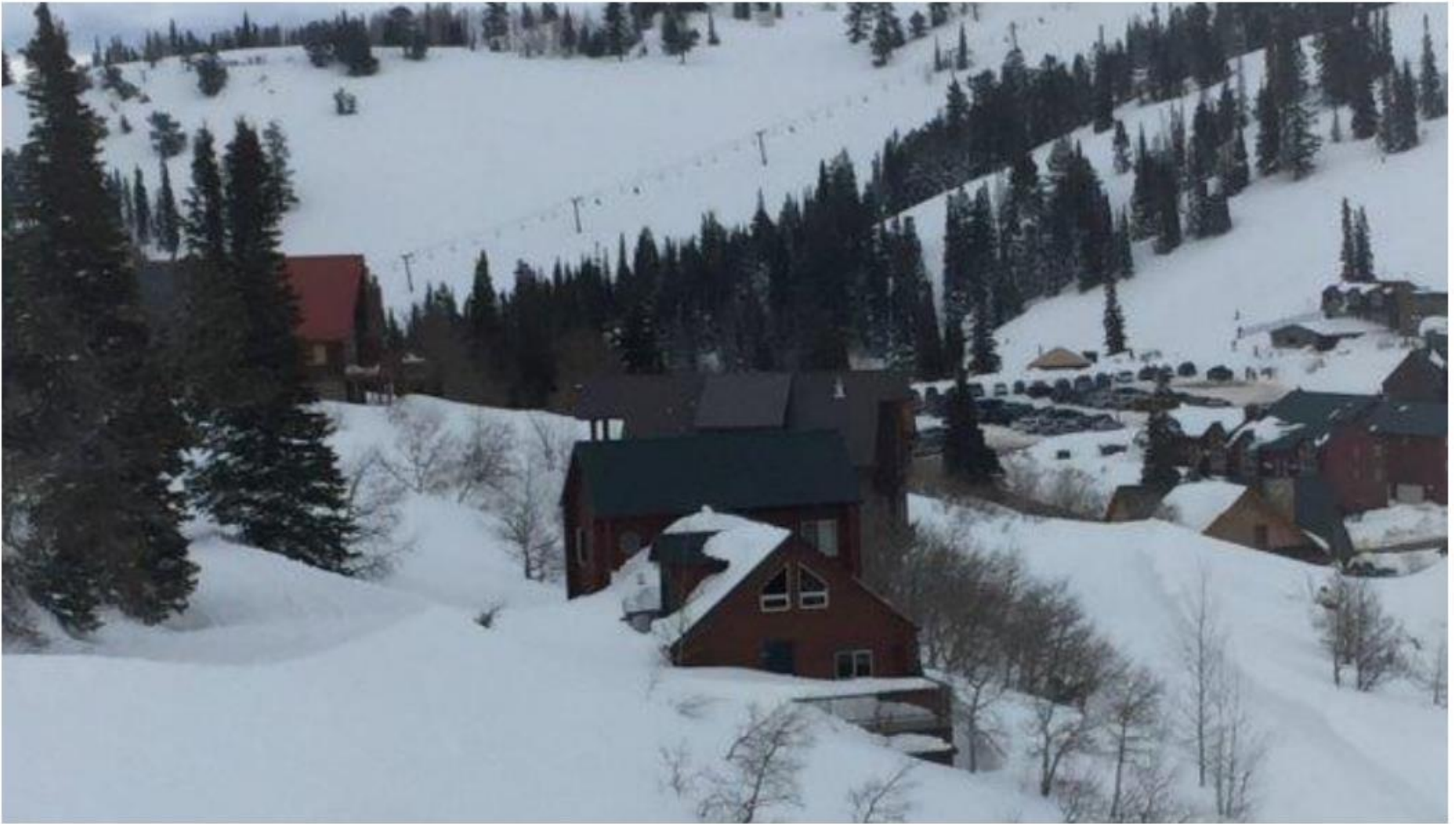
House directly to the east of lot 42. Example of snow load on north side during heavy snow year.
