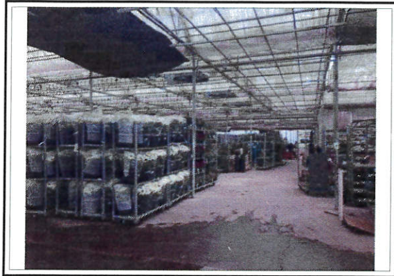
View of Production House
