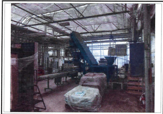
View of Production House
