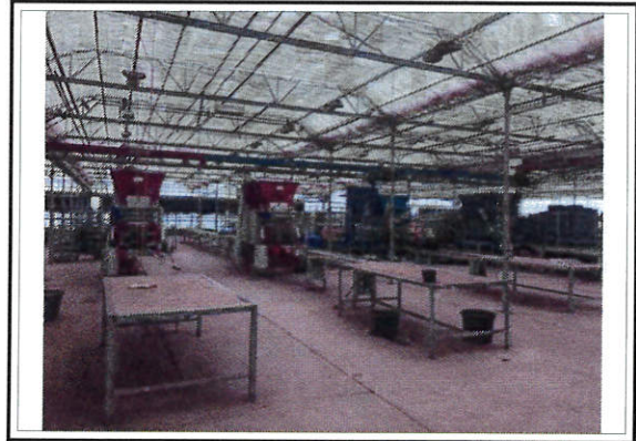
View of Production House
