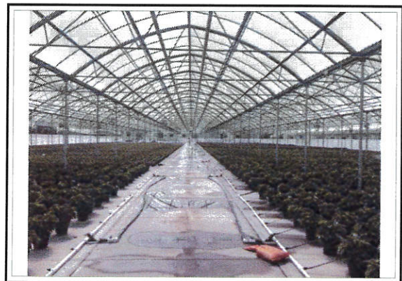
View of S-3 Interior
