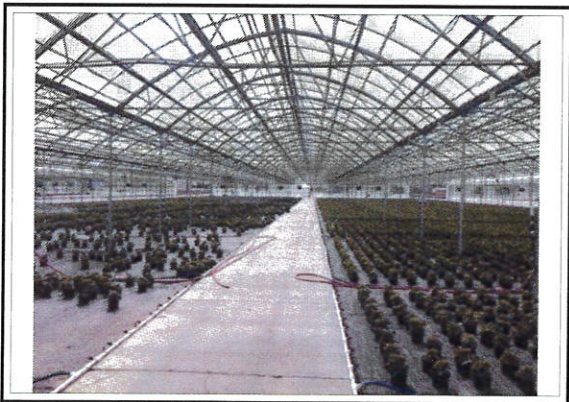
View of S-2 Interior
