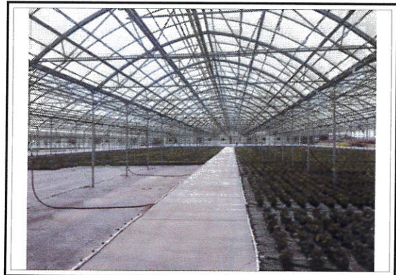
View of S-1 Interior
