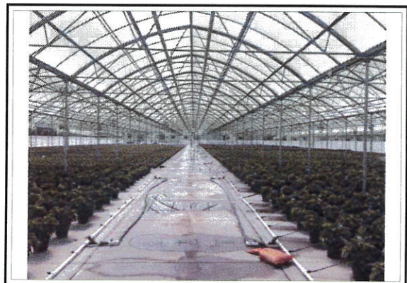
View of S-3 Interior
