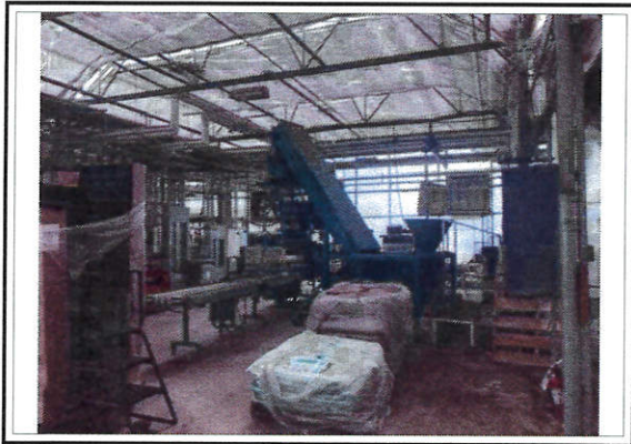
View of Production House
