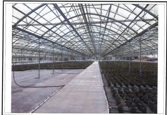
View of S-1 Interior
