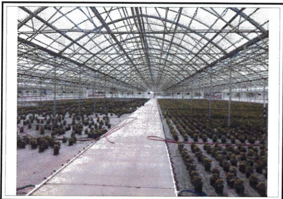
View of S-2 Interior
