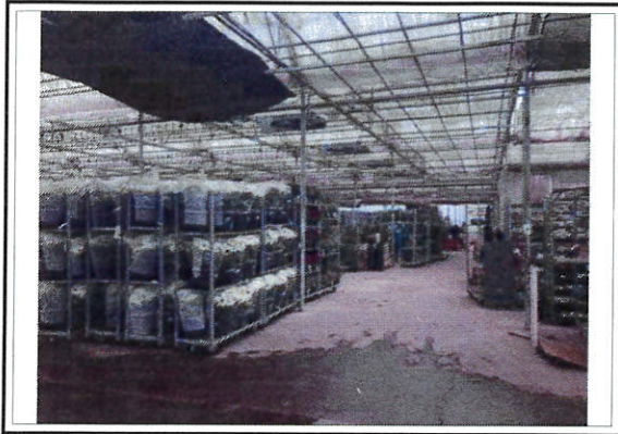
View of Production House
