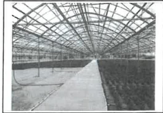
View of S-1 Interior
