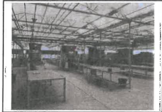
View of Production House
