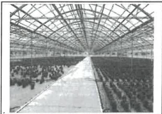
View of S-2 Interior
