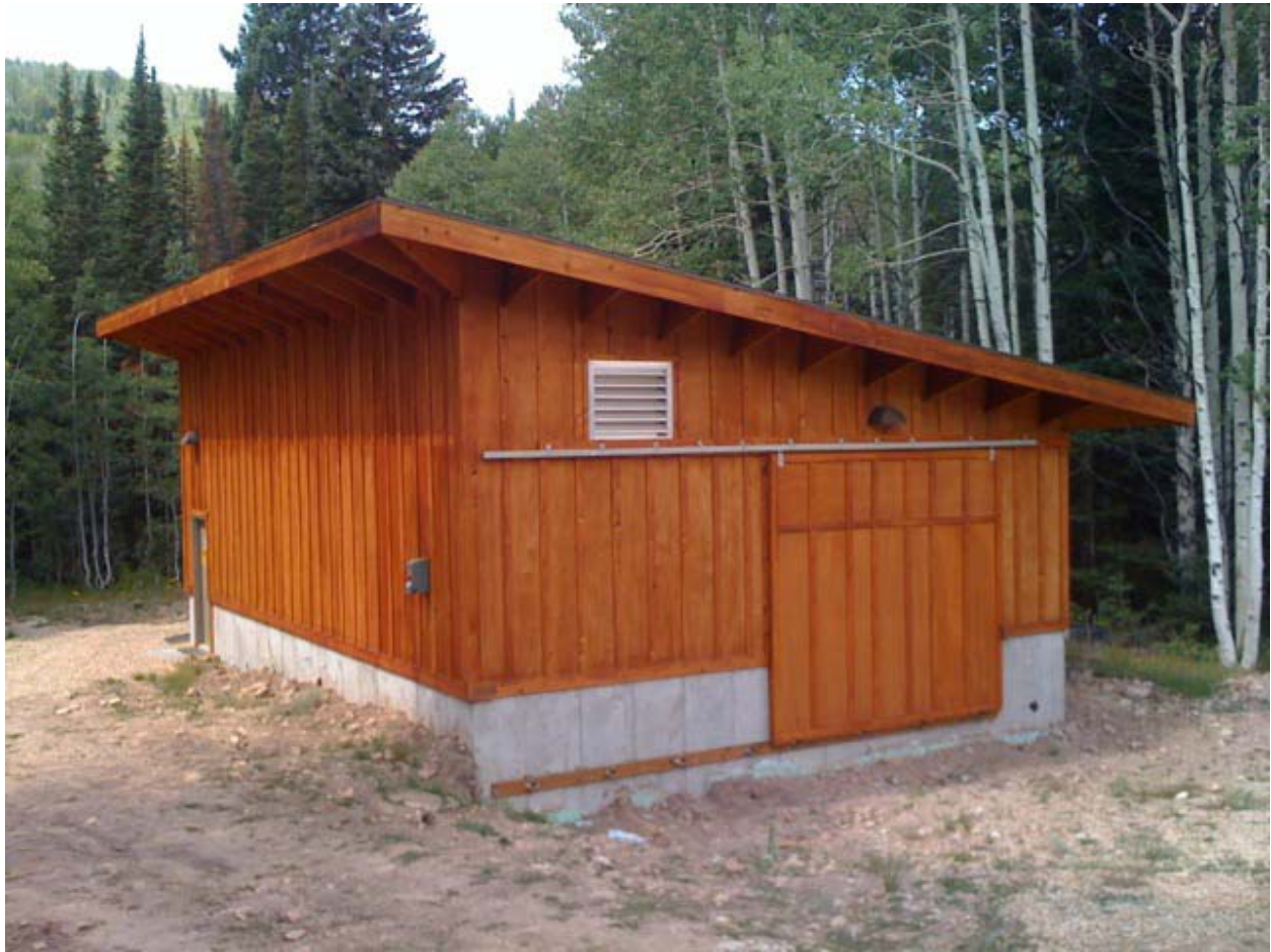
PHOTO OF SIMILAR TYPE BUILDING
