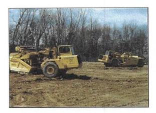
Land grading involves reshaping the ground surface to planned grades as determined by an engineering survey, evaluation, and layout. Land grading provides more suitable topography for buildings, facilities, and other land uses and helps to control surface runoff, soil erosion, and sedimentation during and after construction.
