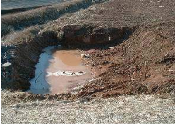
Sediment traps are used to collect sediment-laden runoff from disturbed areas on construction sites
