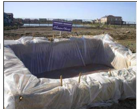
An example of a self-installed concrete washout structure
