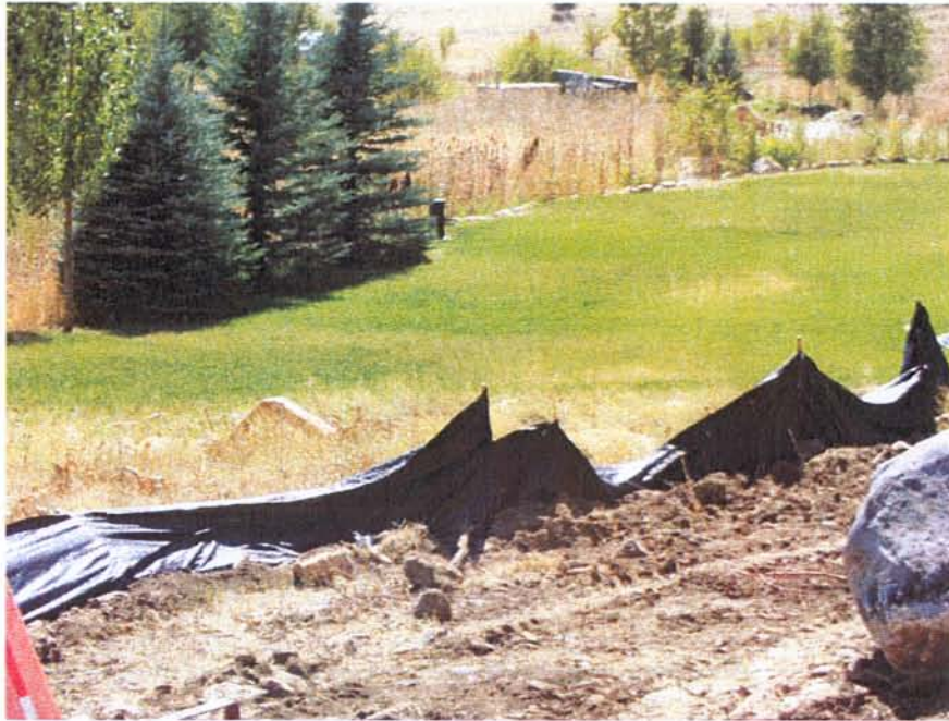
Silt Fence in need of repair
