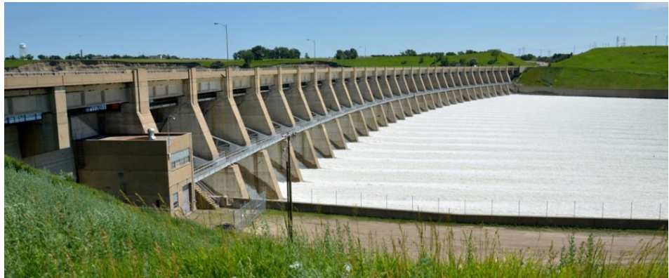
The Garrison Dam on Lake Sakakawea, North Dakota
