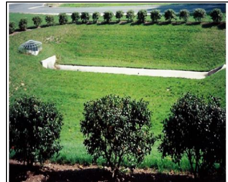
Photo of a dry detention pond designed to temporarily detain runoff during storm events.
