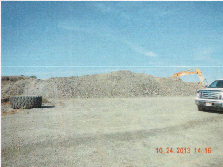
Remaining rock stockpile with trackhoe for loading
