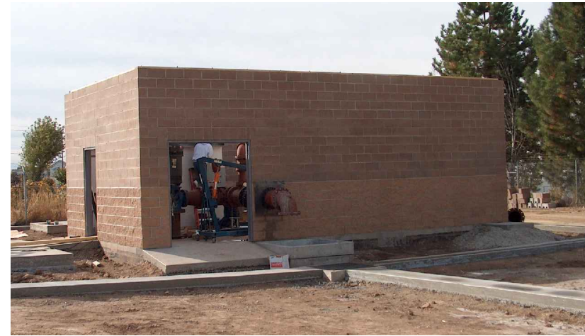
EXISTING WELL HOUSE DURING CONSTRUCTION (NEW PUMP STATION TO BE FINISHED SIMILAR TO EX WELL HOUSE)
