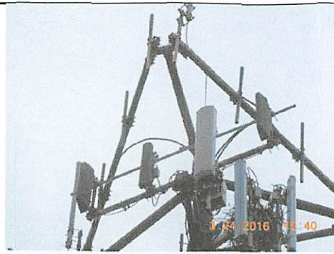
EXISTING ANTENNA ARRAY
