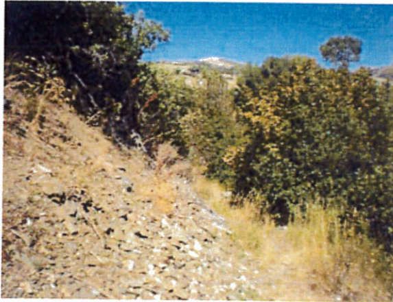
#1 View of roadcut exposed geologic materials comprising the slopes at the site.
