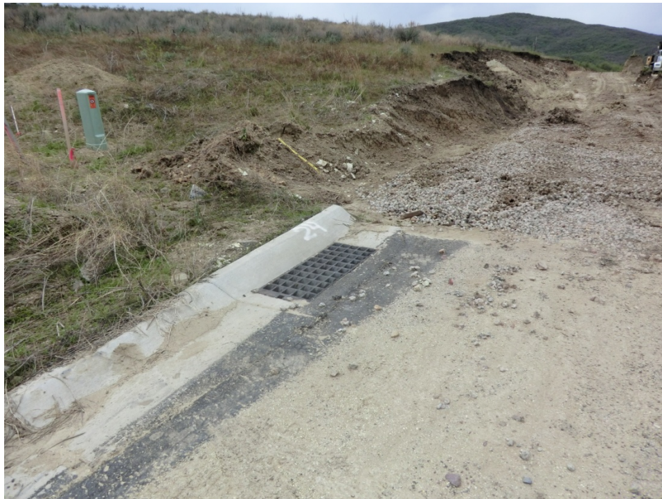
This was the Catch Basin that was a concern
