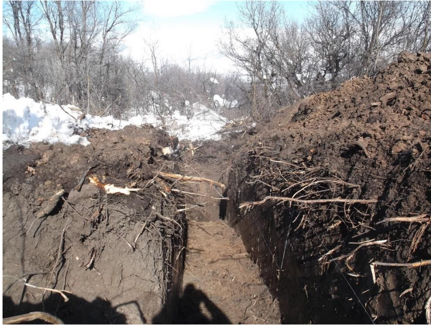
Trench 2, view to south
