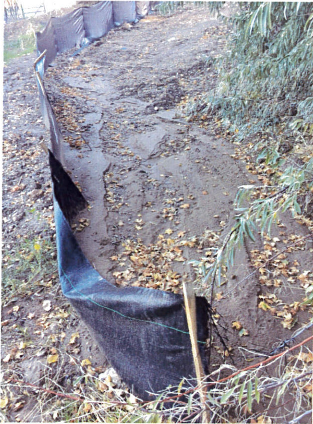
Silt fence requires maintenance
