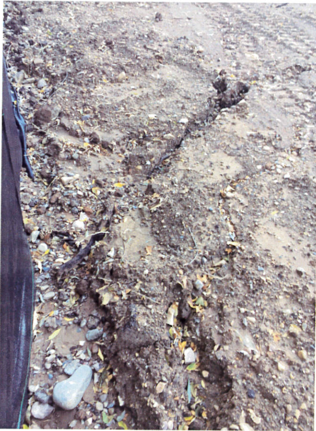
Disturbed areas are eroding and require final stabilization measures to be implemented ASAP
