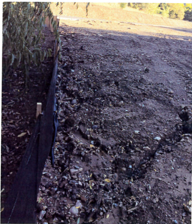
Disturbed areas are eroding and require final stabilization measures to be implemented ASAP
