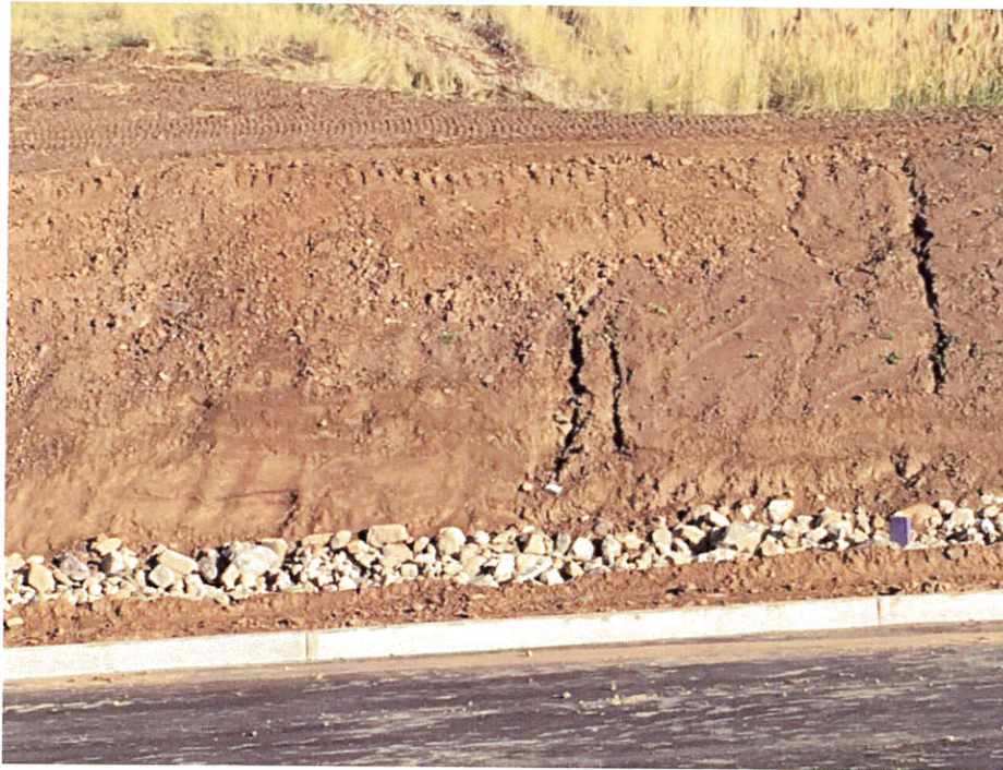
Disturbed areas are eroding and require final stabilization measures to be implemented ASAP
