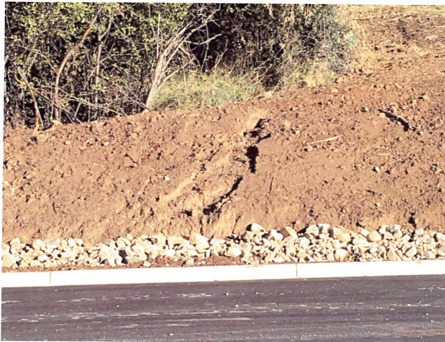
Disturbed areas are eroding and require final stabilization measures to be implemented ASAP
