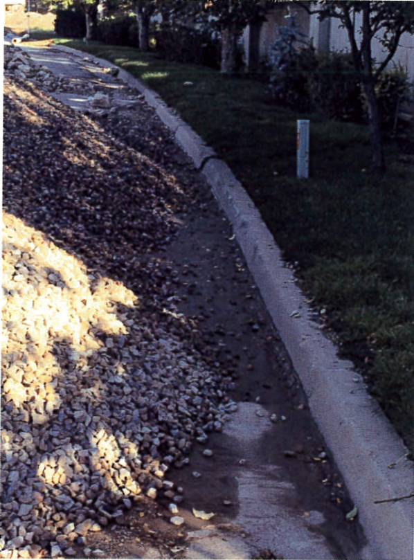
Sediment and soil deposits need to be cleaned up ASAP
