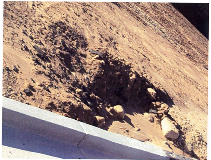
Disturbed areas are eroding and require final stabilization measures to be implemented ASAP
