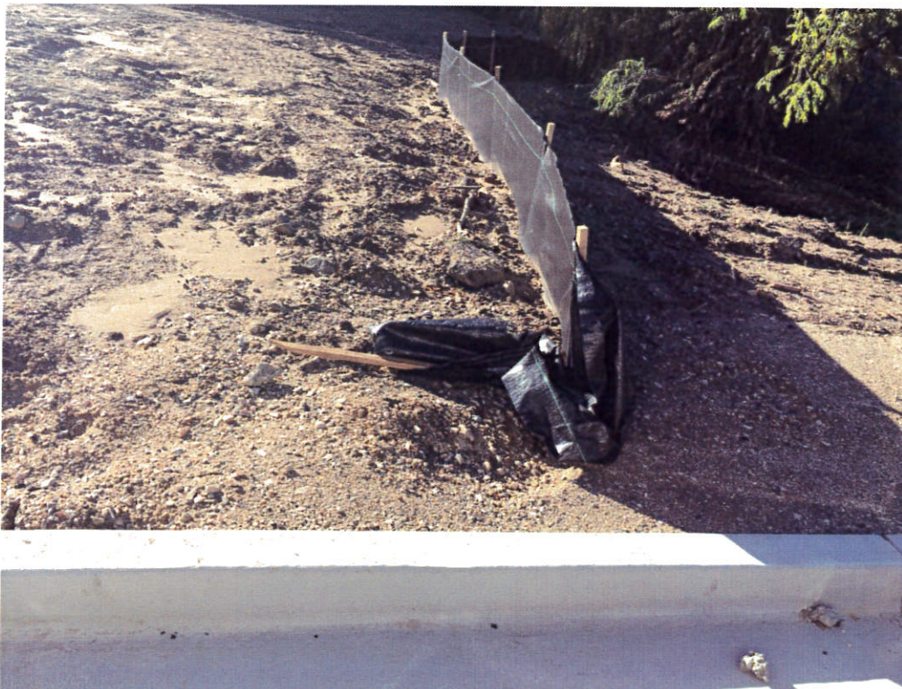
Silt fence requires maintenance
