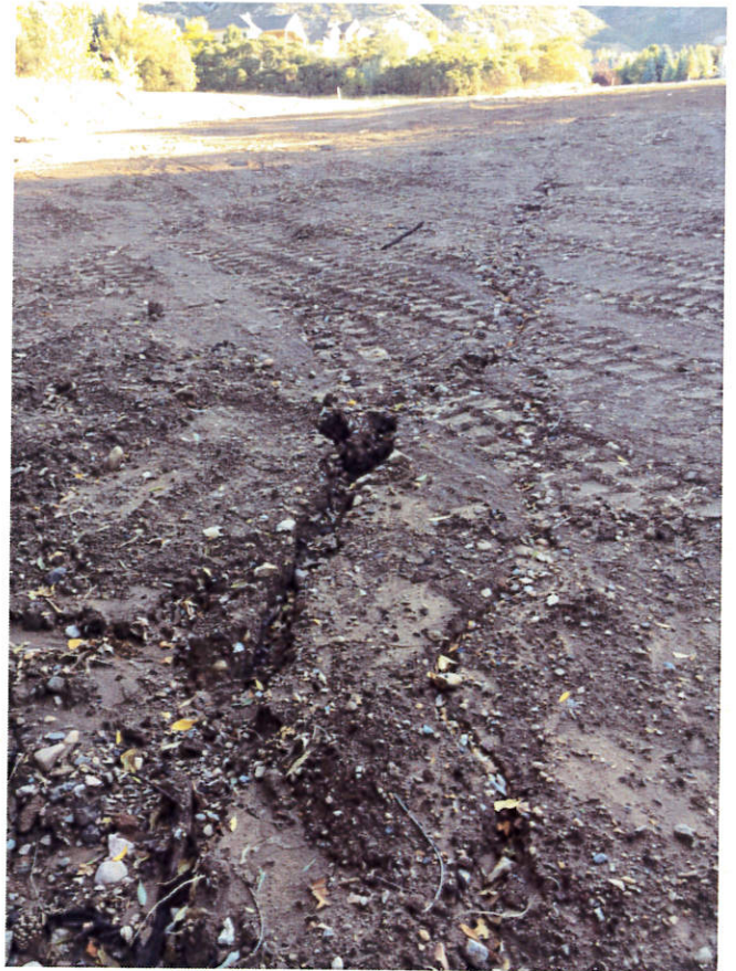
Disturbed areas are eroding and require final stabilization measures to be implemented ASAP
