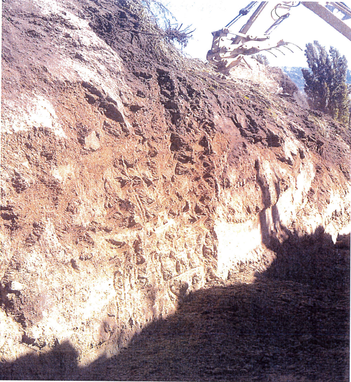
Extension of Test Pit 3- West side of sidewall.
