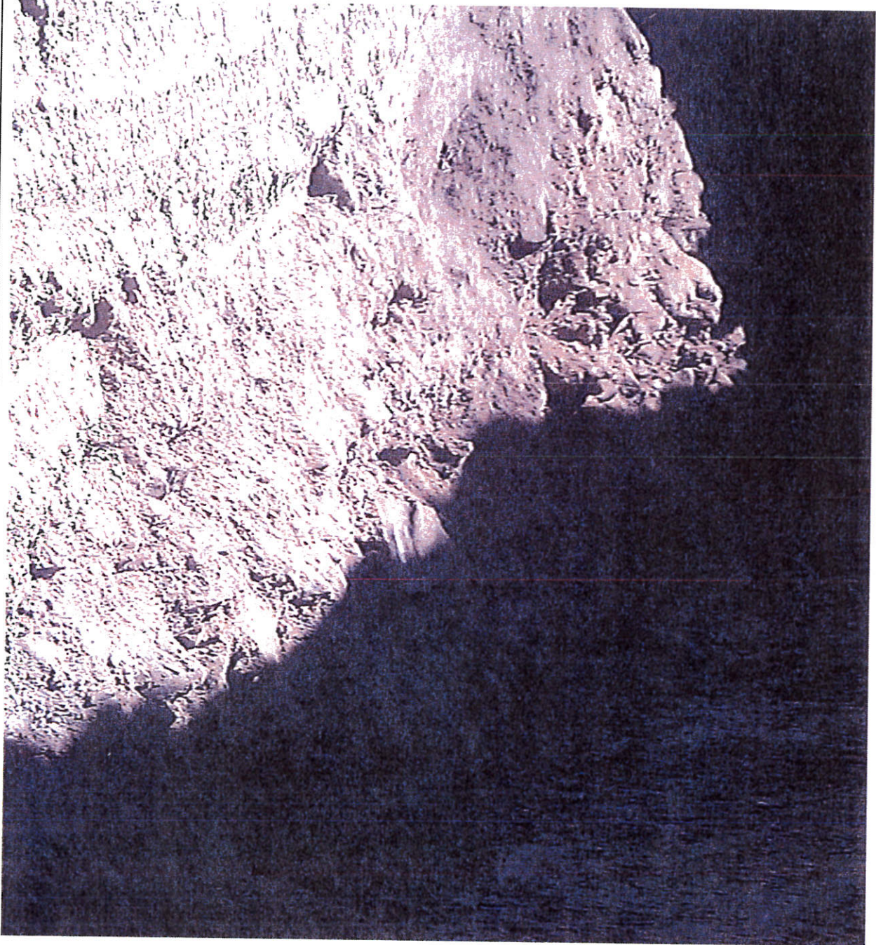
Test Pit 3- West side of sidewall at the north end of the trench. Showing the gravel in the sidewall.
