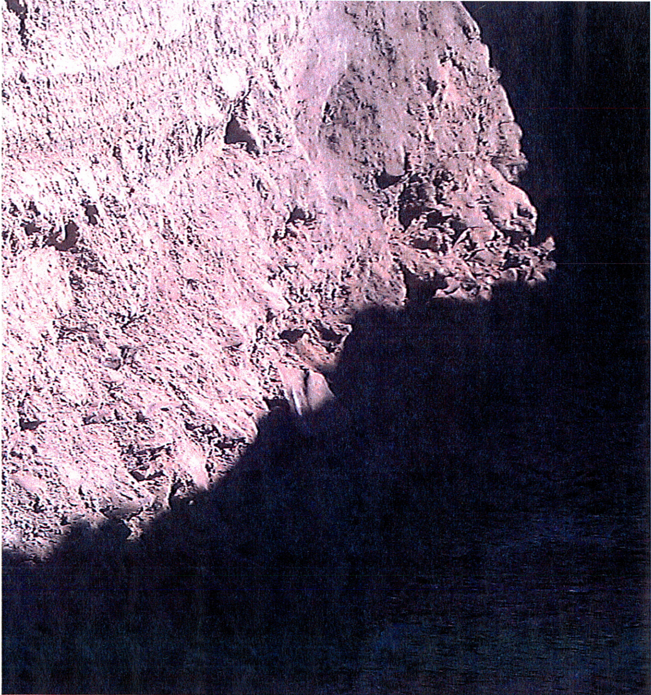
Test Pit 3- West side of sidewall at the north end of the trench. Showing the gravel in the sidewall.
