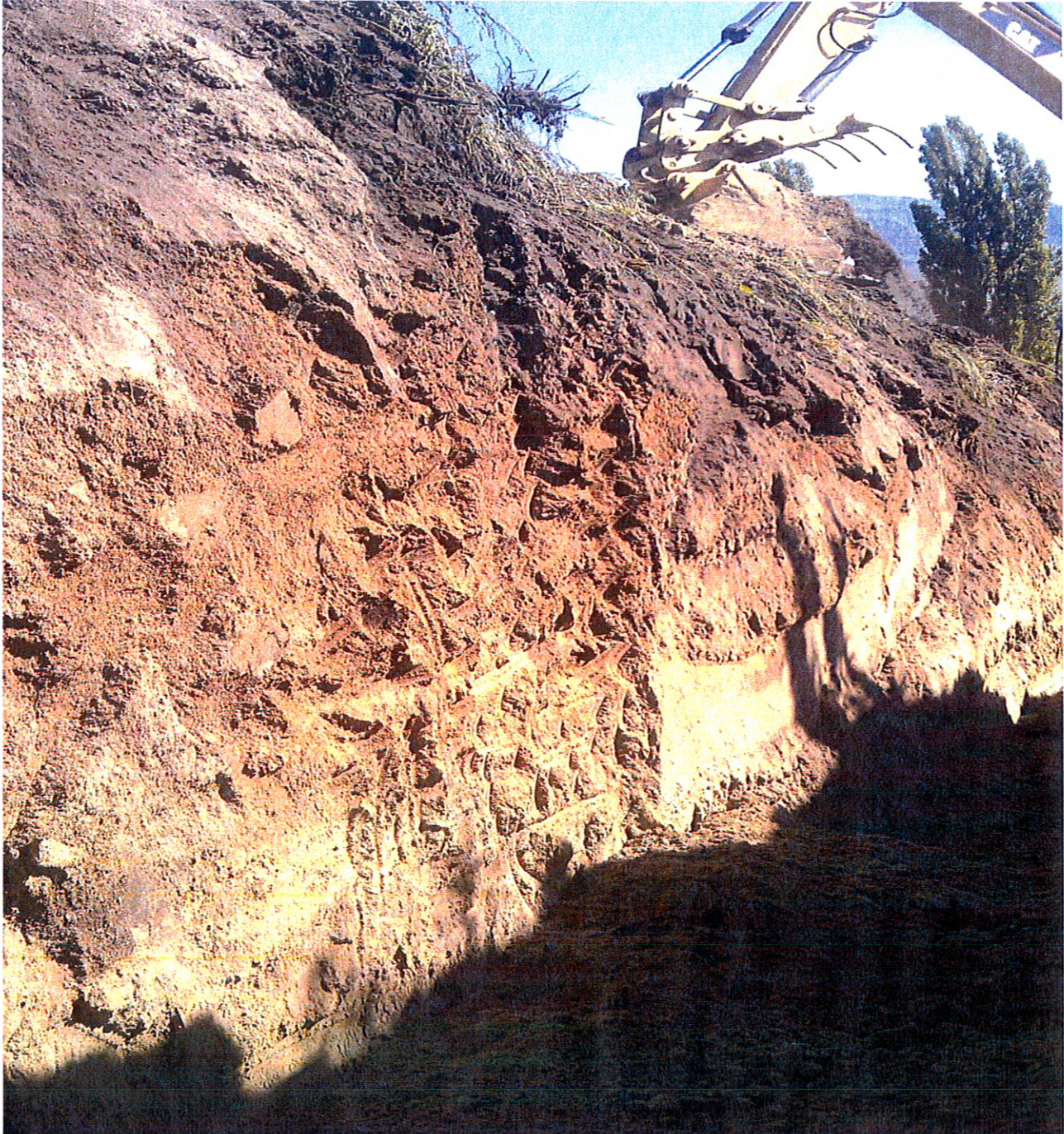
Test Pit 3- West side of sidewall.
