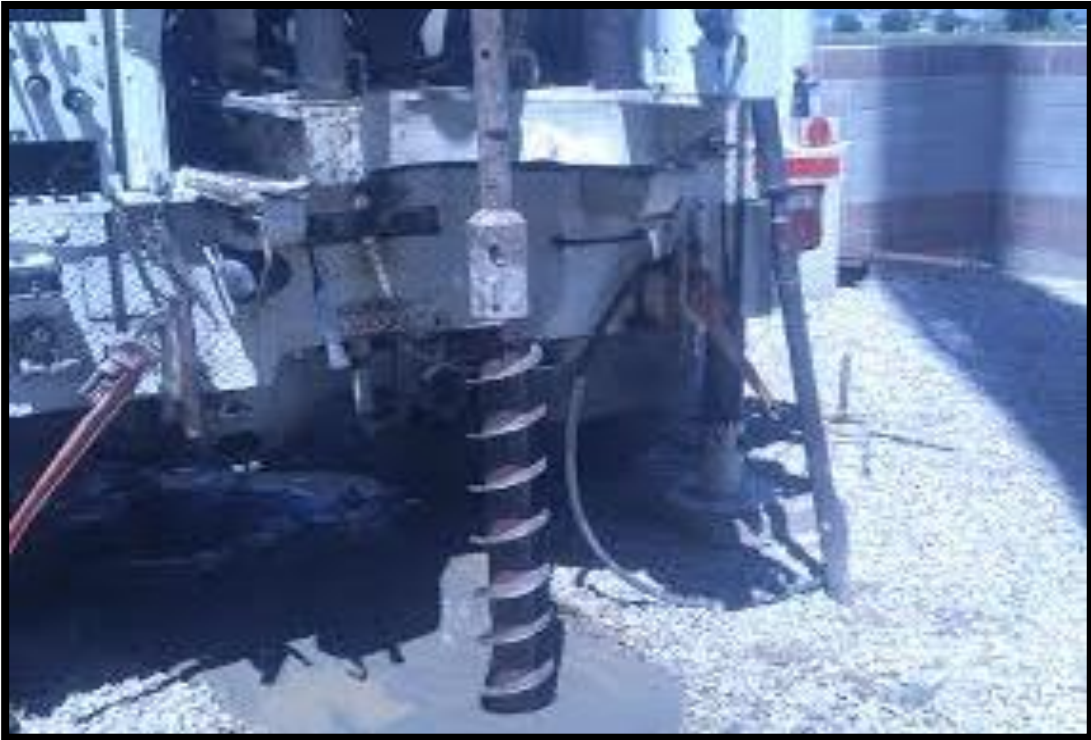
5) DRILL RIG DURING DRILLING
