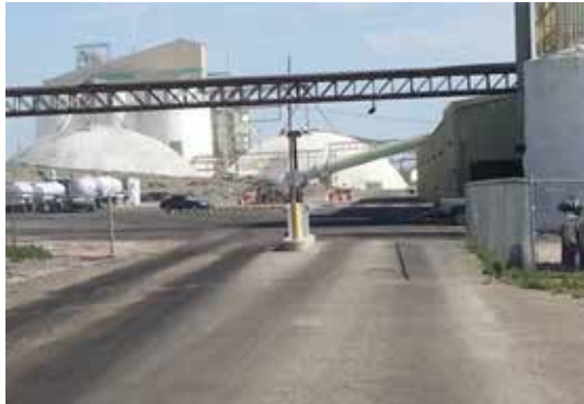
Existing Sign - west of road - new posts and footings
