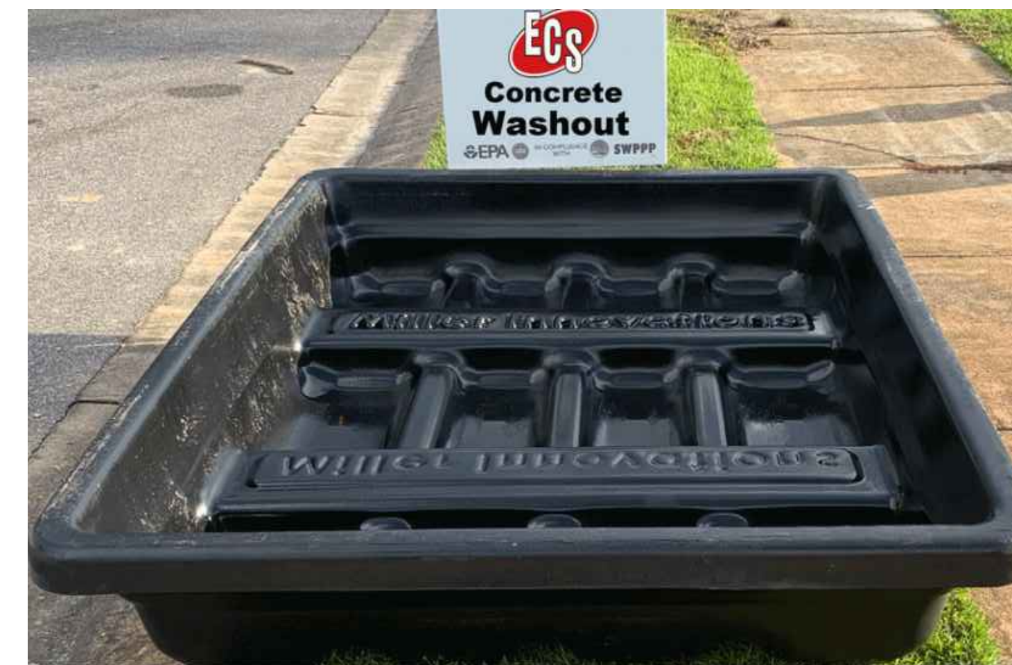
CONCRETE WASHOUT AREA NOT TO SCALE
