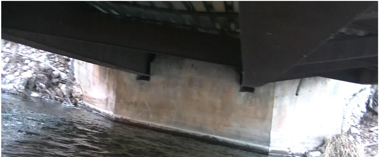
Figure 6. Post-flooding and repair photograph of west bridge abutment.
