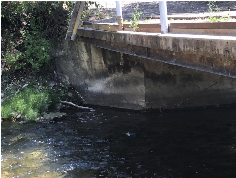
Figure 5. NW bridge abutment on October 12, 2022 looking west (before 2023 flooding).
