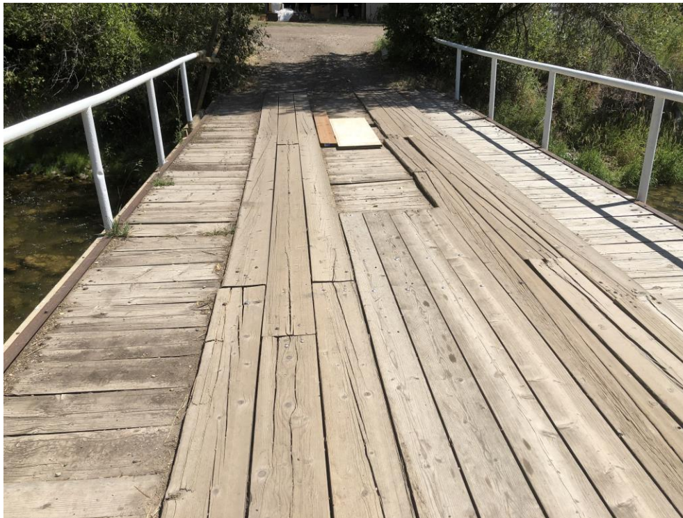
Figure 3. Bridge condition on October 12, 2022 looking west (before 2023 flooding).
