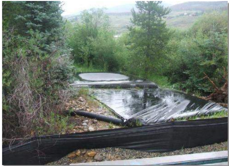
Photograph DW-2. Dewatering bags used for a relatively large dewatering operation.
