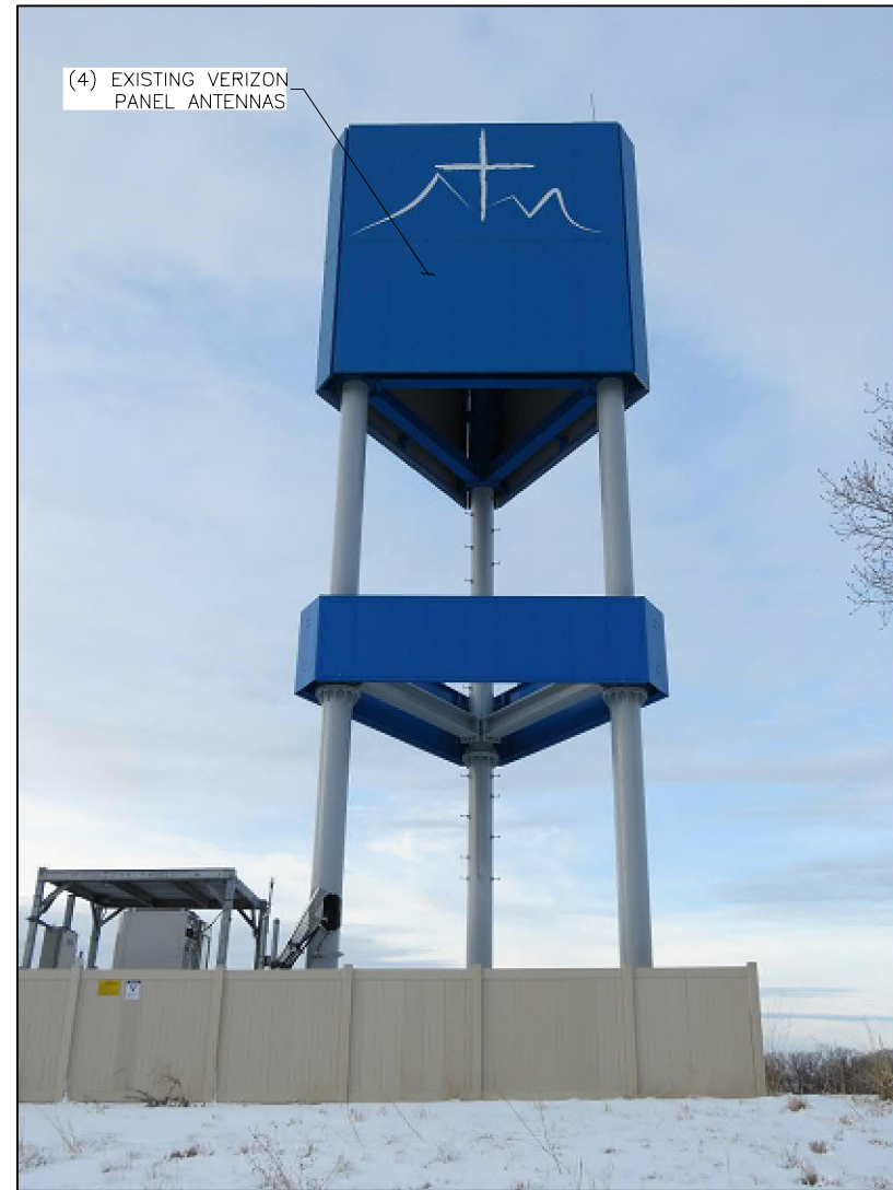
VIEW OF EXISTING TOWER (LOOKING SOUTHWEST)
