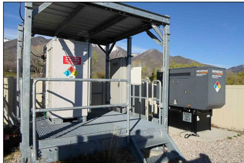
VIEW OF EXISTING EQUIPMENT PLATFORM
