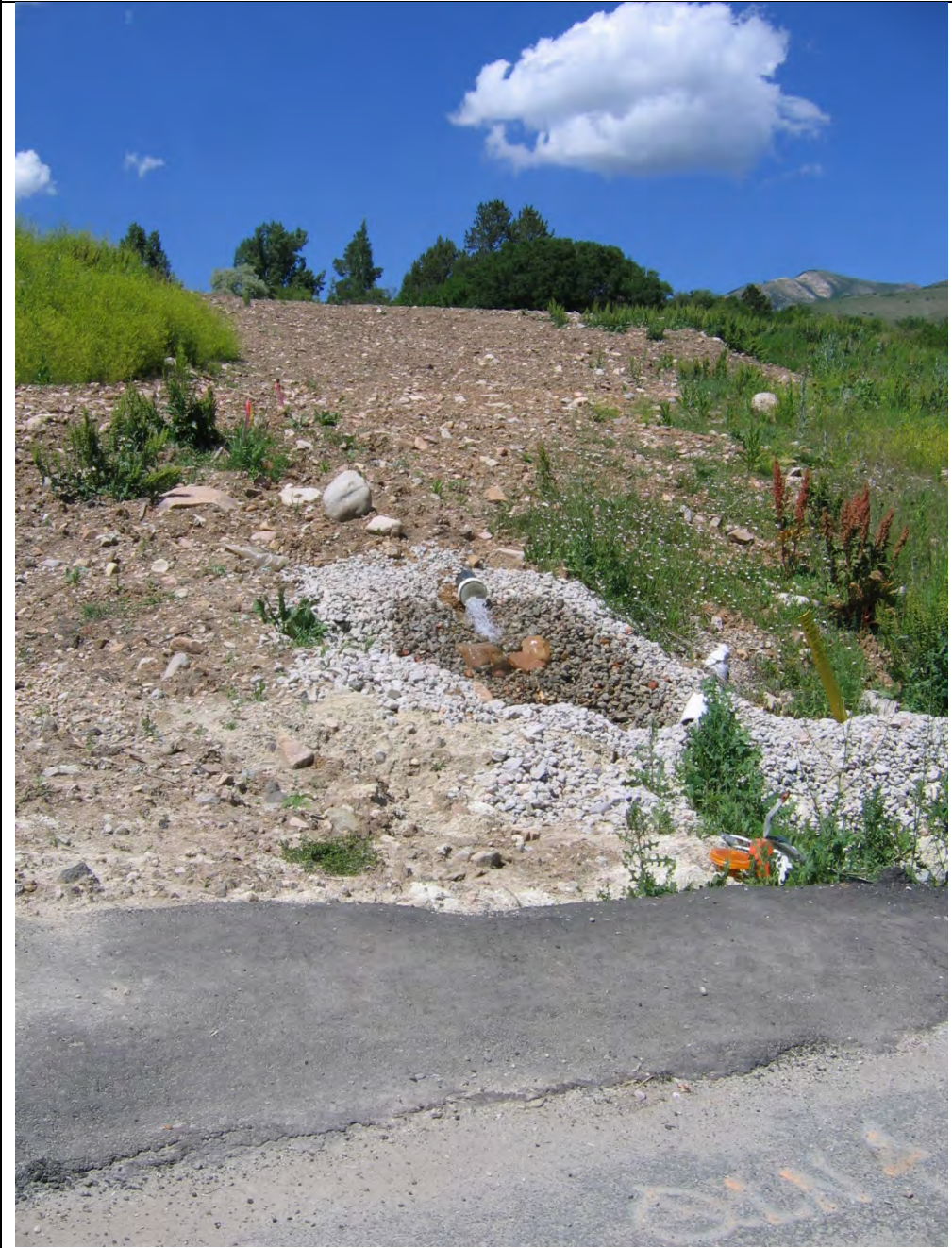
Photo 14. July 2009 UGS site visit. Regraded area with new drain.
