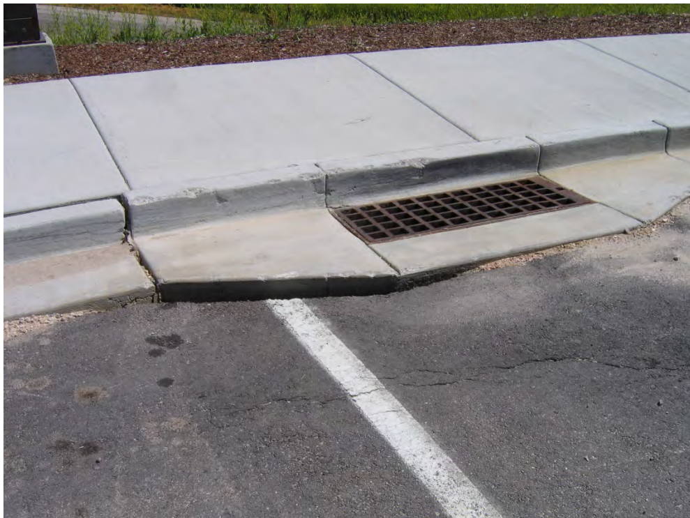
Photo 13. July 2009 UGS site visit. Displacement between gutter and pavement near storm drain.
