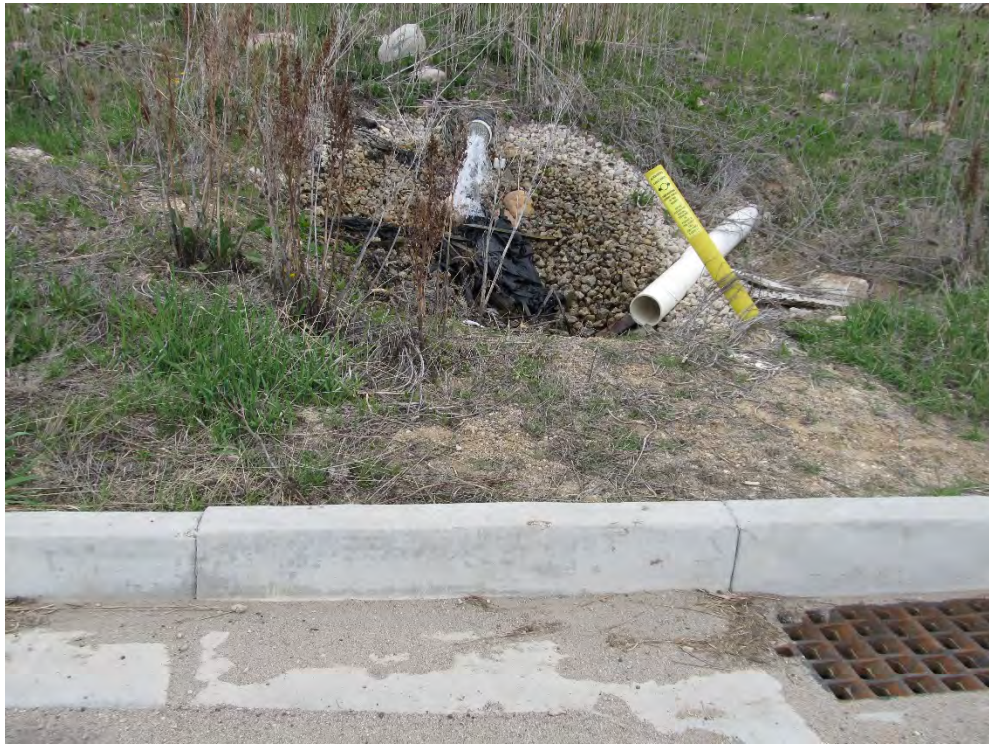
Photo 17. April 2014 UGS site visit. Drain and new curb and gutter.
