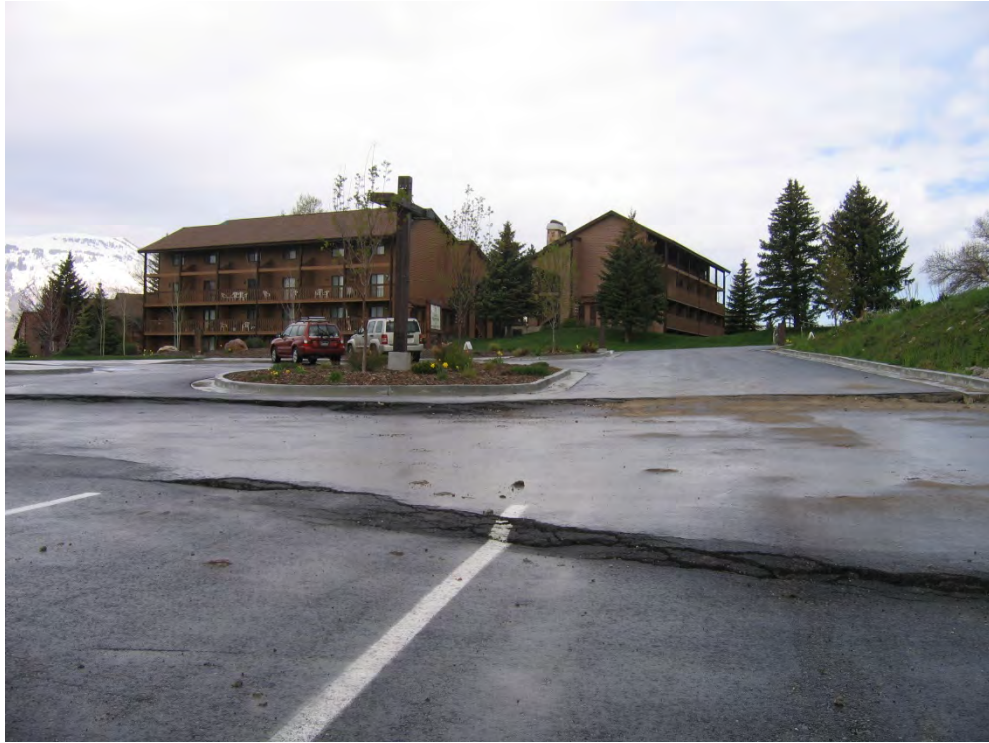
Photo 13. July 2009 UGS site visit. Displacement between gutter and pavement near storm drain.
