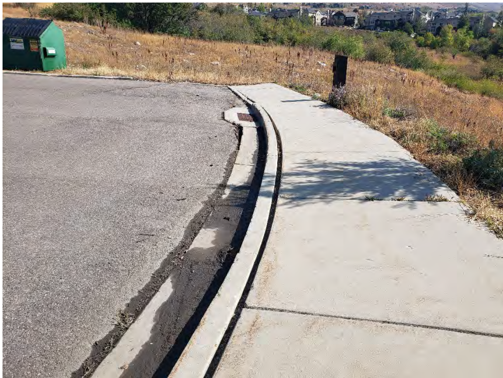
Photo 30. Pull apart between curbing and sidewalk. Compare to Photo 19.
