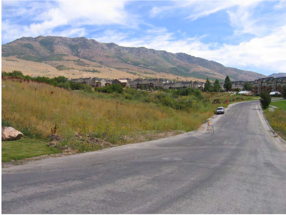
Photo 7. August 2008 UGS site visit. Landslide toe at Moose Hollow Drive.
