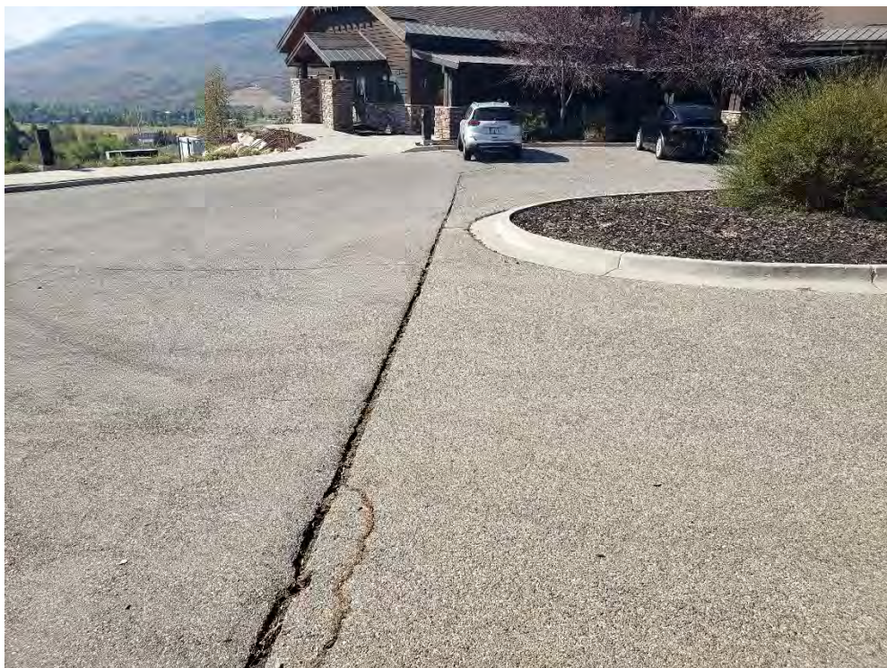
Photo 28. Saw cut pavement repair.
