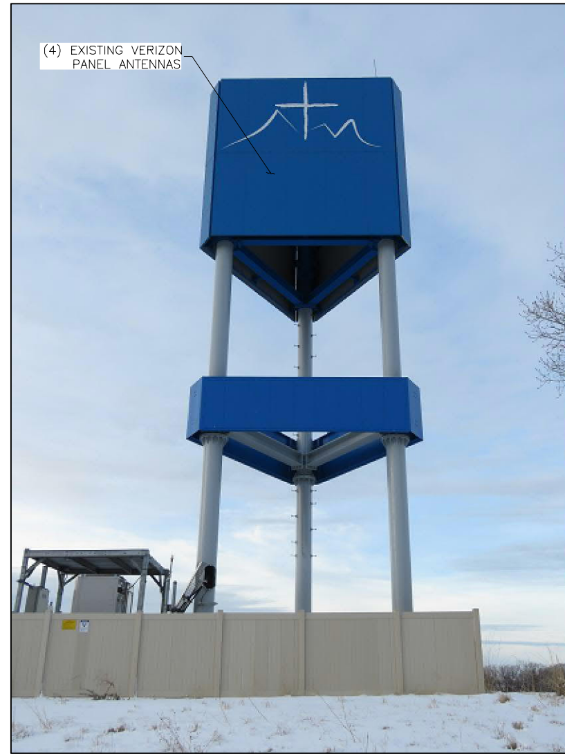
VIEW OF EXISTING TOWER (LOOKING SOUTHWEST)
