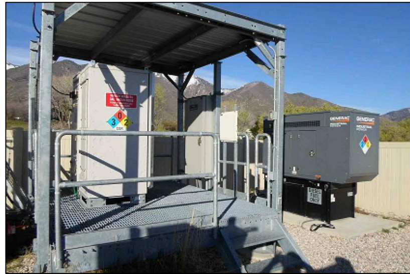
VIEW OF EXISTING EQUIPMENT PLATFORM
