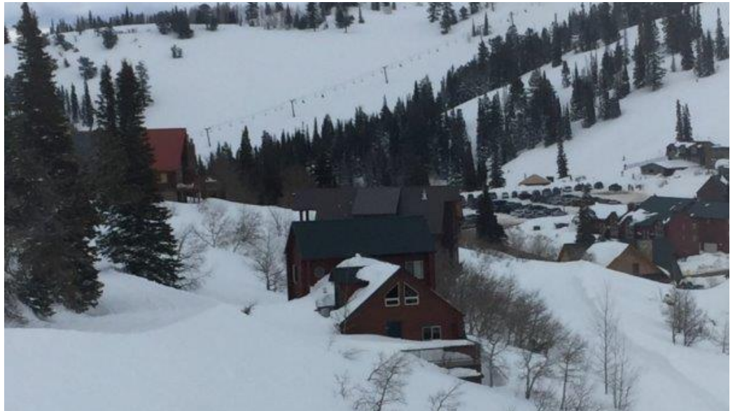
House directly to the east of lot 42. Example of snow load on north side during heavy snow year.
