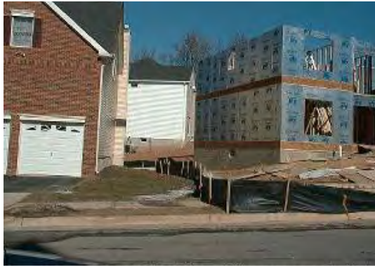
In sequenced construction, sites are completed in stages and completed portions are permanently stabilized before other areas are disturbed
