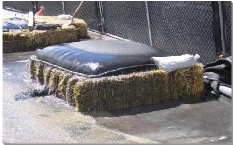
Photograph DW-1. A relatively small dewatering operation using straw bales and a dewatering bag.
