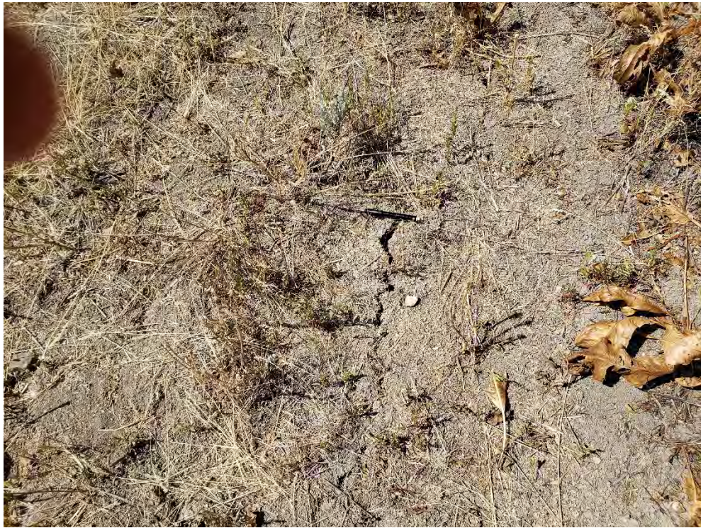
Photo 5. Possible expansive soil cracking.
