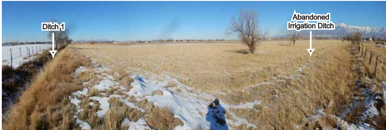
Photo 21. Northeast view of Ditch 1 and abandoned irrigation ditch taken from southeast corner of the Project Area. The abandoned irrigation ditch had no OHWM indicators present and was dominated by upland plant communities during the December 29, 2020 site inspection.
