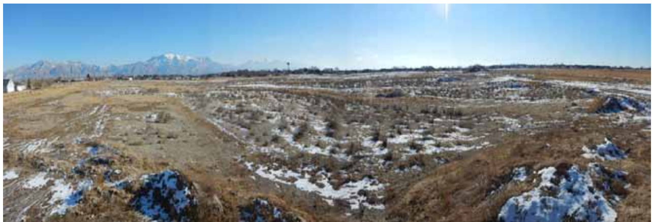
Photo 7. Southeast view of upland area recently filled and graded.
