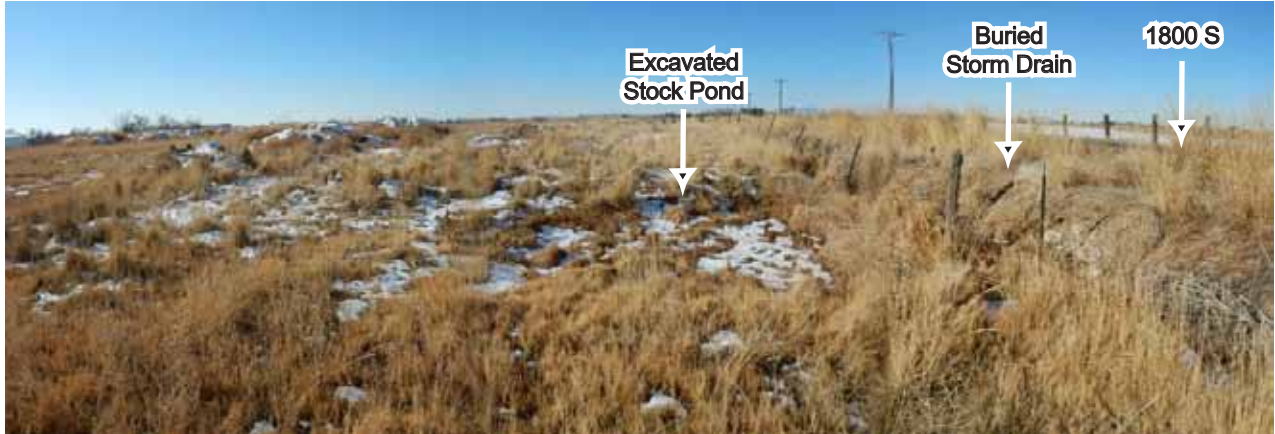
Photo 2. West view of remnants of an excavated stock pond located near the northeast corner of the Project Area. Wetland plants have established on the bottom of the excavated pond. Water was observed in stock pond during December 29, 2020 site inspection. Buried storm drain also pictured.
