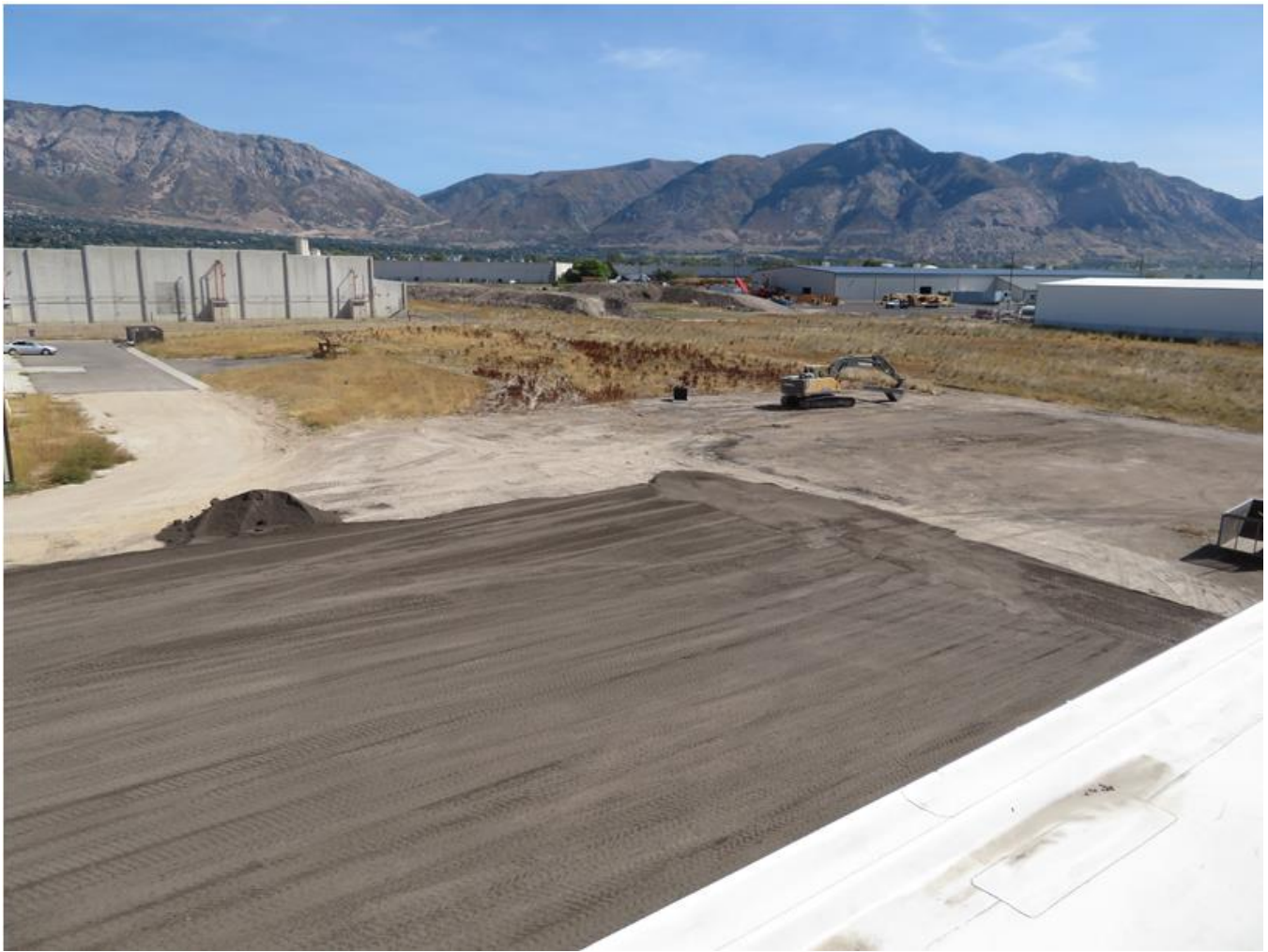
View from the roof of proposed facility
