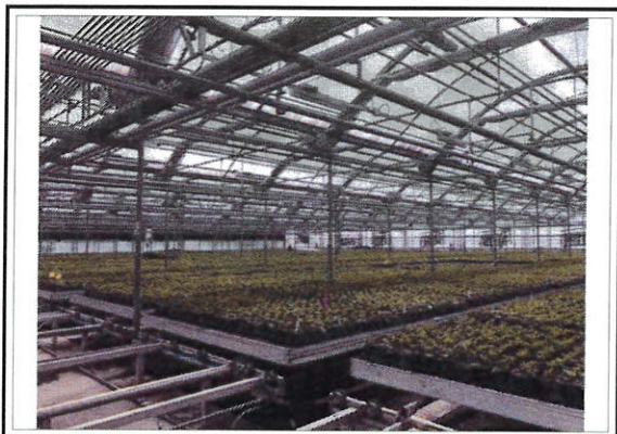
View of Table House
