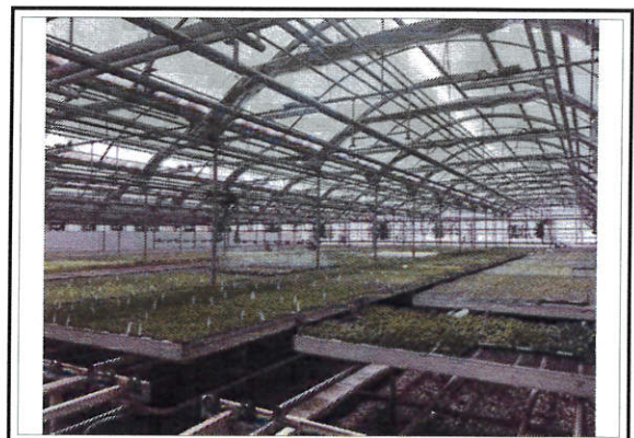
View of Table House
