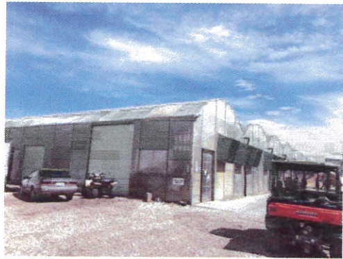
View of Greenhouse
