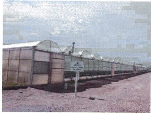
View of Greenhouse
