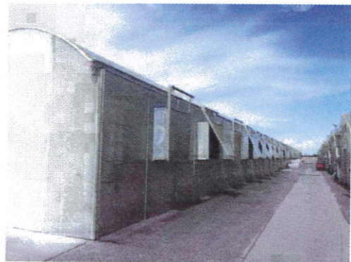
View of Greenhouse
