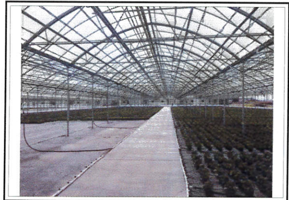
View of S-1 Interior
