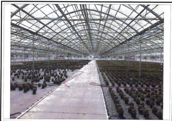
View of S-2 Interior
