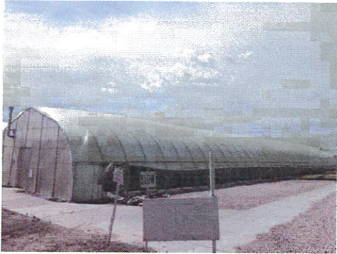
View of Greenhouse
