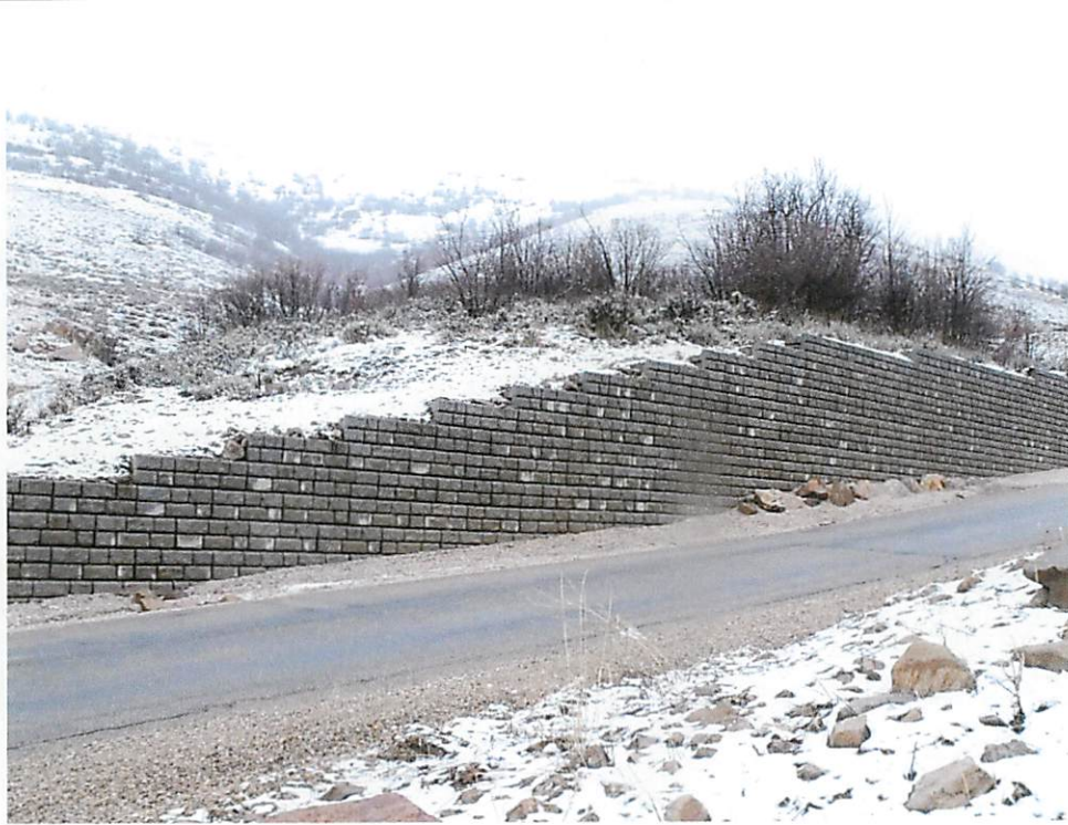
Photo 1. Retaining wall on Maple Drive
