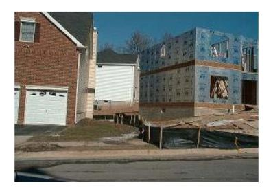
Construction sequencing is a specified work schedule that coordinates the timing of land-disturbing activities and the installation of erosion and sediment control measures. Construction site phasing involves disturbing only part of a site at a time to prevent erosion from dormant parts. Grading activities and construction are completed and soils are effectively stabilized on one part of the site before grading and construction commence at another part.
