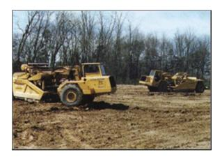
Land grading involves reshaping the ground surface to planned grades as determined by an engineering survey, evaluation, and layout. Land grading provides more suitable topography for buildings, facilities, and other land uses and helps to control surface runoff, soil erosion, and sedimentation during and after construction.
