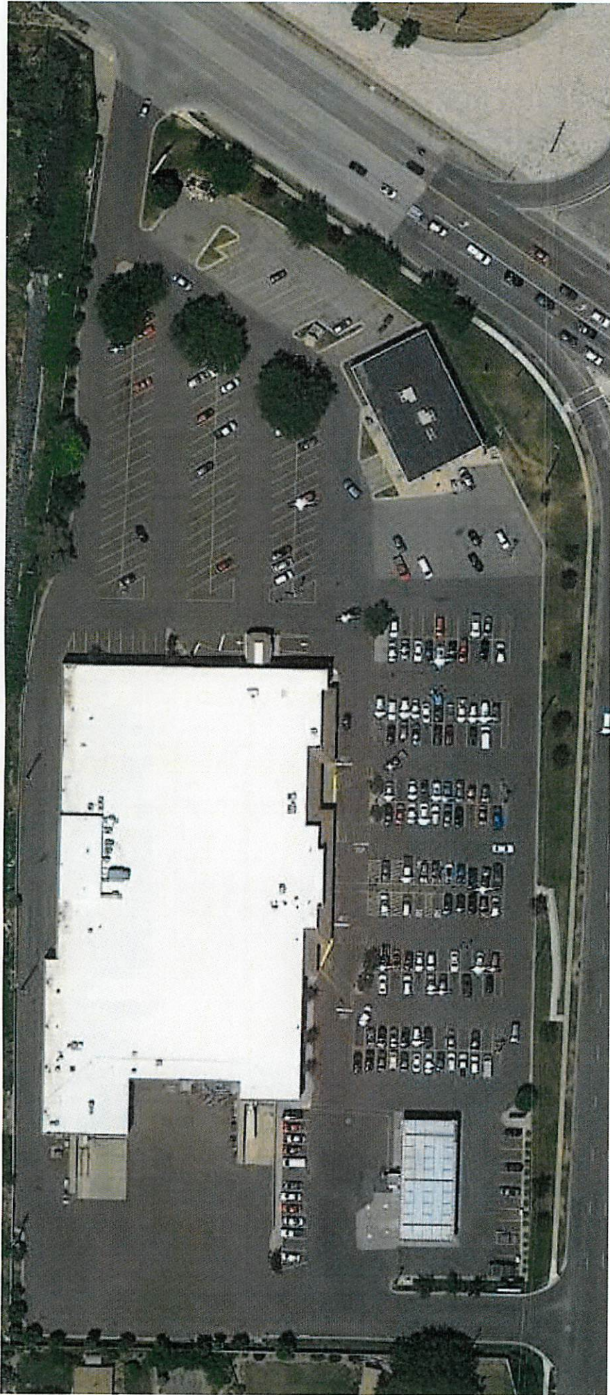
Smiths Grocery at 12th and Harrison. Approximately five acres with a 62,000 square foot grocery store, 4,400 square feet of other retail, and a gas canopy.
