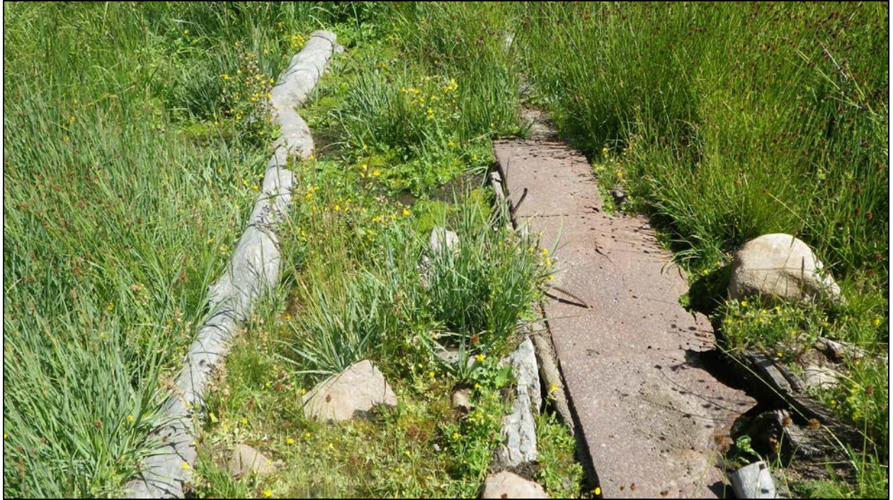
Steel plate over the old spring head area at larger wetland.
