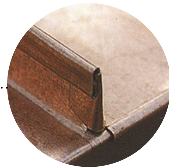
ROOF CORTEN STANDING SEAM
