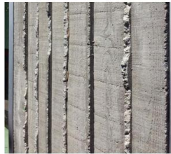
Concrete Foundation: vertical formwork, rough finish
