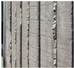
Concrete Foundation: vertical formwork, rough finish
