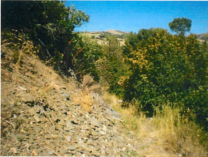
#1 View of roadcut exposed geologic materials comprising the slopes at the site.
