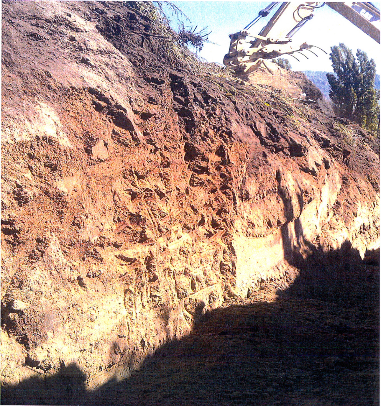
Extension of Test Pit 3- West side of sidewall.
